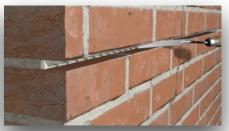
The next step is to fill the groove with a first layer of mortar about 10 mm thick and place a pre-cut anchor in it.
